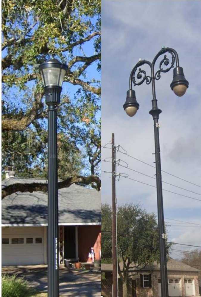
Existing Light Poles
